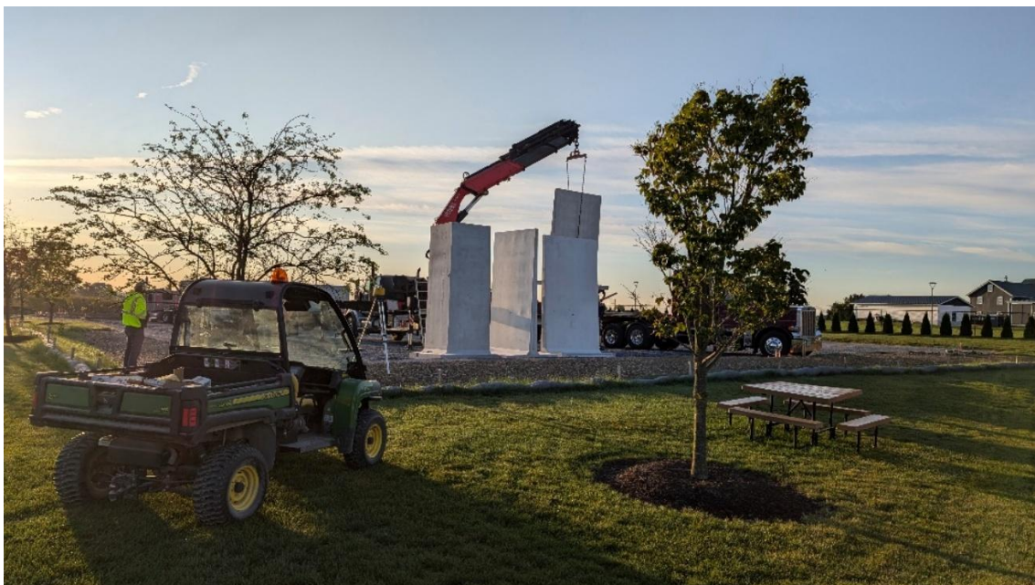
Yard Waste Site Walls Construction
