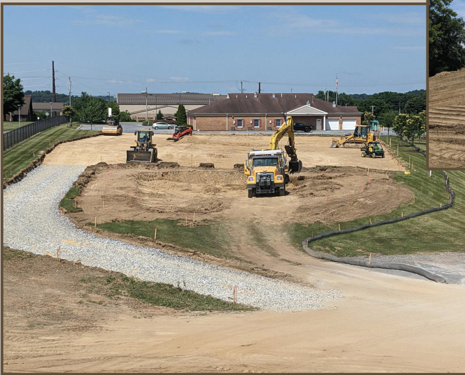
Left: Construction of stormwater basin and yard waste facility.
